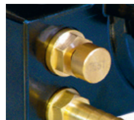
Test feature for routine testing
